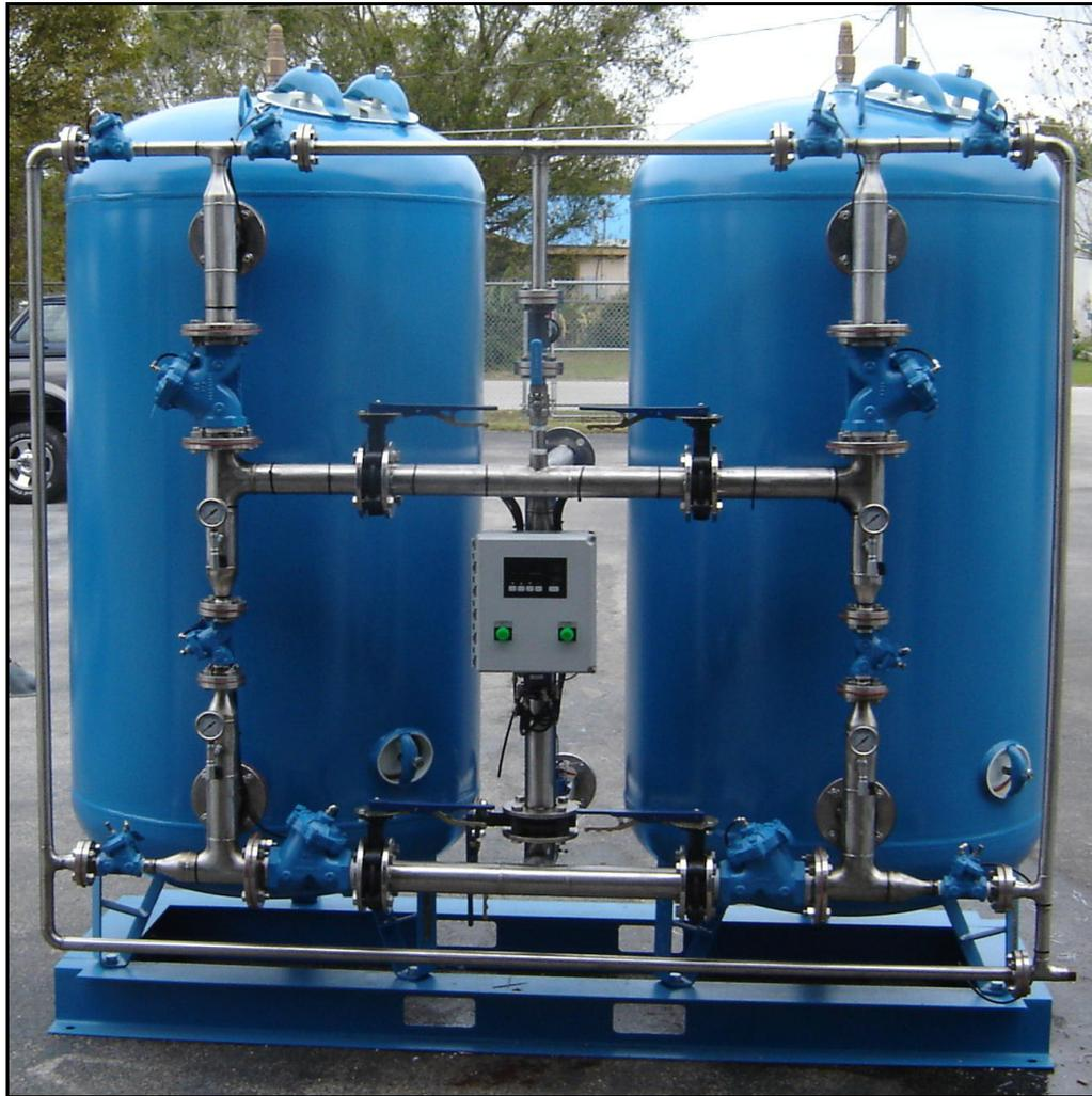
The ASD-3660-3/1/SS is one of our most popular softeners. The ASD-3660-3/1/SS features 1" regeneration and 3" outlet stainless steel face piping, a twin alternating stager and controller which can be controlled with air or water pressure, a flow sensor, and optional flow transmitter capabilities as well as many other features.
